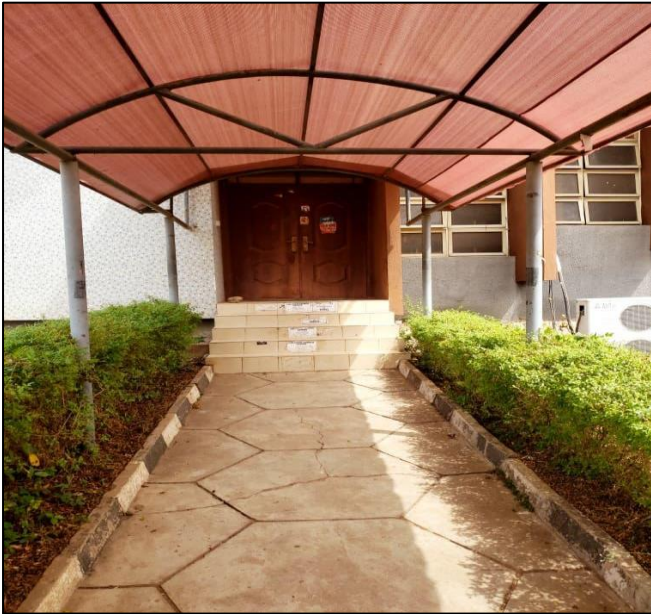
Fig 8 Main Entrance Door to the Lecture Theatre at the Faculty of Social Sciences Showing Measured Door Width and Steps at Selected Entry Points. (Source: Field Survey, 2026).
