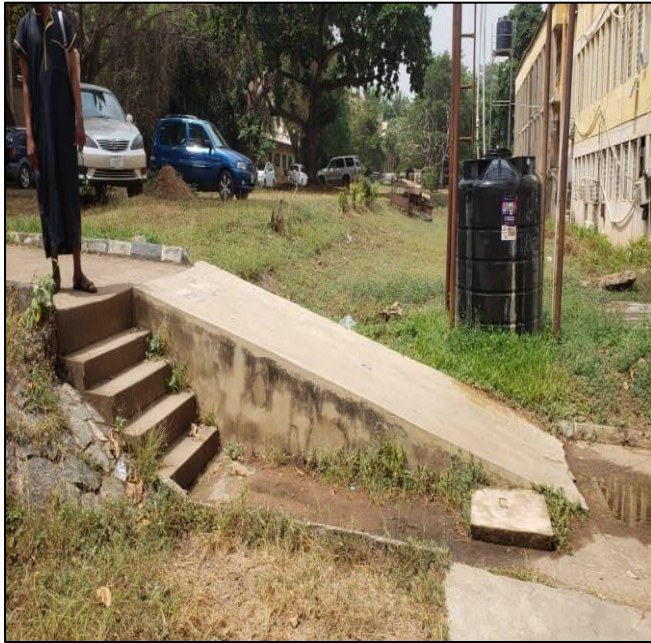
Fig 4 Faculty of Education Secondary Ramp Showing Measured Width and Slope. (Source: Field Survey, 2026)
