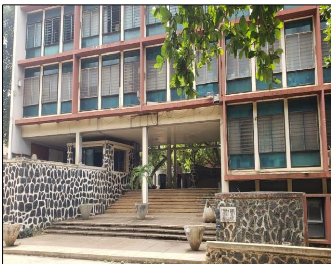
Fig 5 Faculty of Arts Entrance Showing the Absence of a Ramp. (Source: Field Survey, 2026).
