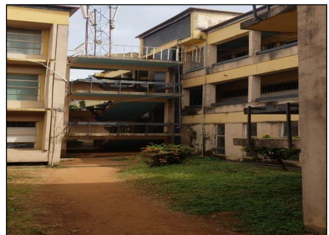
Fig 18 and 19 Staircase at the Faculty of Education Showing Measured Tread and Riser Dimensions. (Source: Field Survey, 2026).
