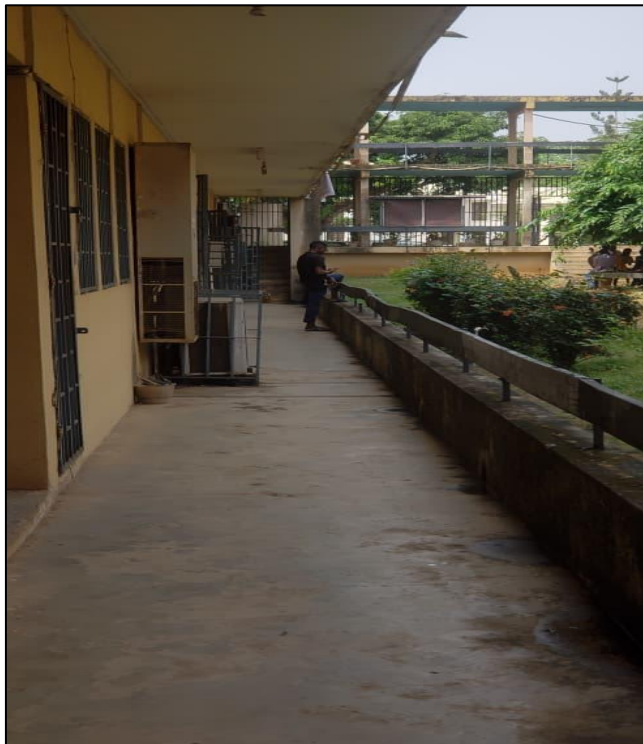
Fig 12 and 13 Internal Corridor at the Faculty of Education Showing Measured Circulation Width. (Source: Field Survey, 2026).
