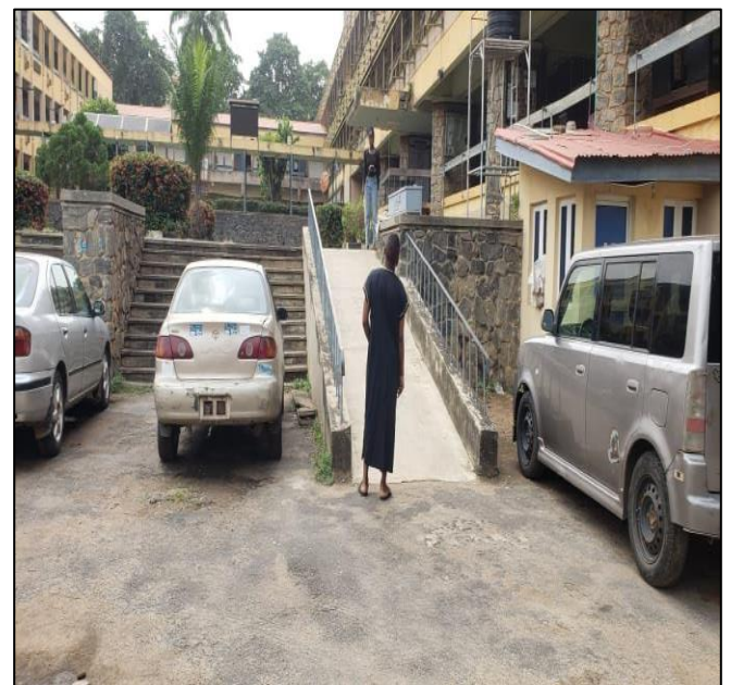
Fig 3 Entrance Ramp at the Faculty of Education Showing Measured Width, Rise, and Length (Source: Field Survey, 2026)
