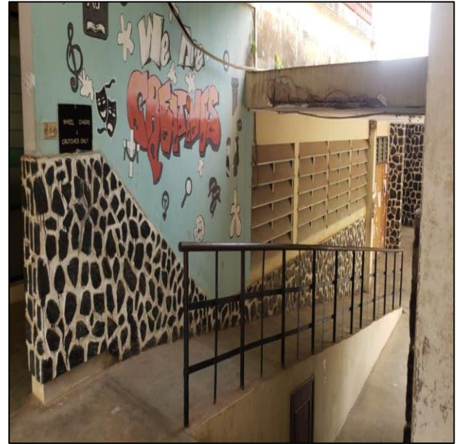
Fig 6 Faculty of Arts Secondary Ramp Showing Measured Width and Slope. (Source: Field Survey, 2026).
