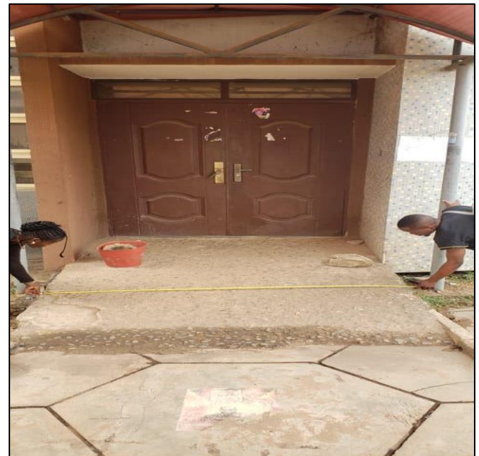
Fig 2 Faculty of Social Sciences Secondary Ramp Showing Measured Width and Slope. (Source: Field Survey, 2026).
