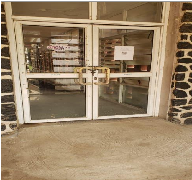
Fig 9 Main Lecture Theatre Entrance Door at the Faculty of Education. (Source: Field Survey, 2026).
