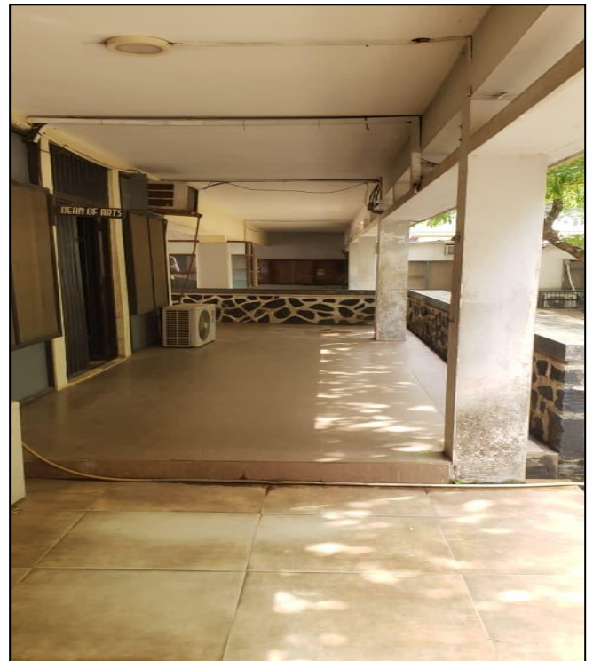
Fig 14 and 15 Internal Corridor at the Faculty of Arts Showing Circulation Width. (Source: Field Survey, 2026).
