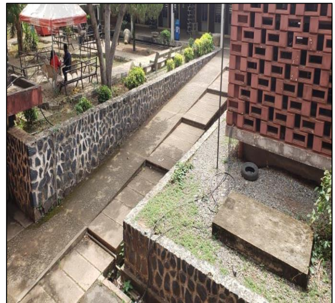
Fig 7 Faculty of Arts Secondary Ramp Showing Measured Width and Slope. (Source: Field Survey, 2026).
