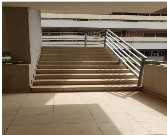
Fig 16 and 17 Main Staircase at the Faculty of Social Sciences Showing Tread, Riser, and Width Dimensions. (Source: Field Survey, 2026).
