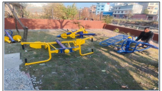
Fig 5 Installation of Exercise Equipment at Open Spaces Along Riverside
