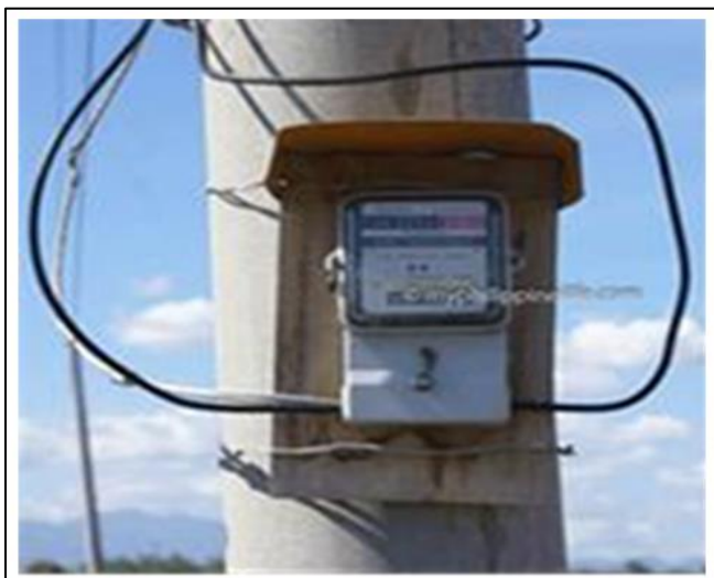
Fig 3 Pole-Mounted Smart Prepaid Meter
