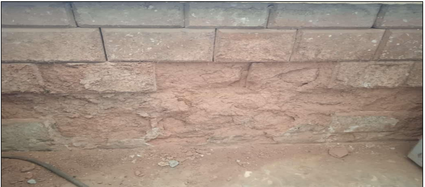
Plate 1: Deteriorated CSEBs Wall
