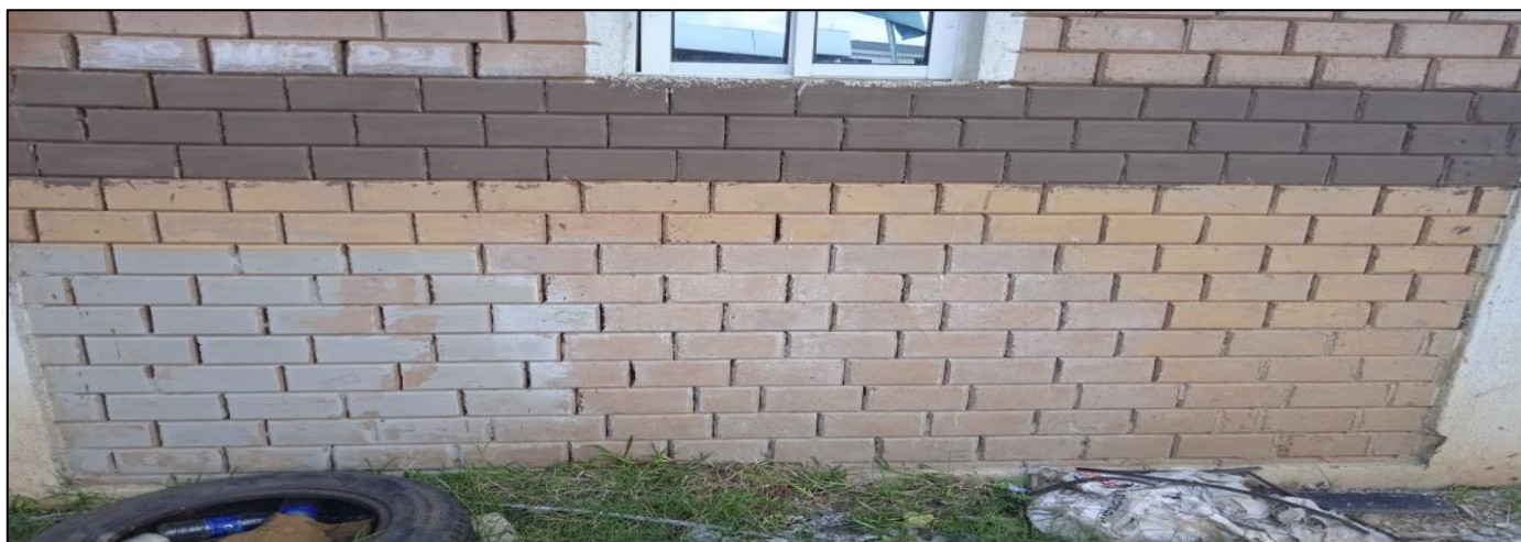
Plate 10: Observation of Samples after Three (3) Months of Polishing the CSEBs Wall Surface
