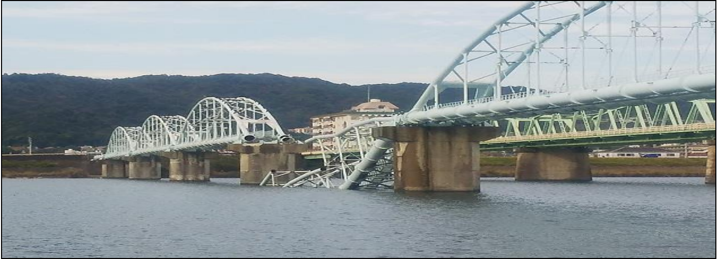
Fig 1 Wakayama Aqueduct Bridge Failure
