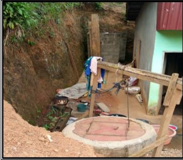
Photo 3: Wells Built in Melen 6 Photo Essomba, 2020
