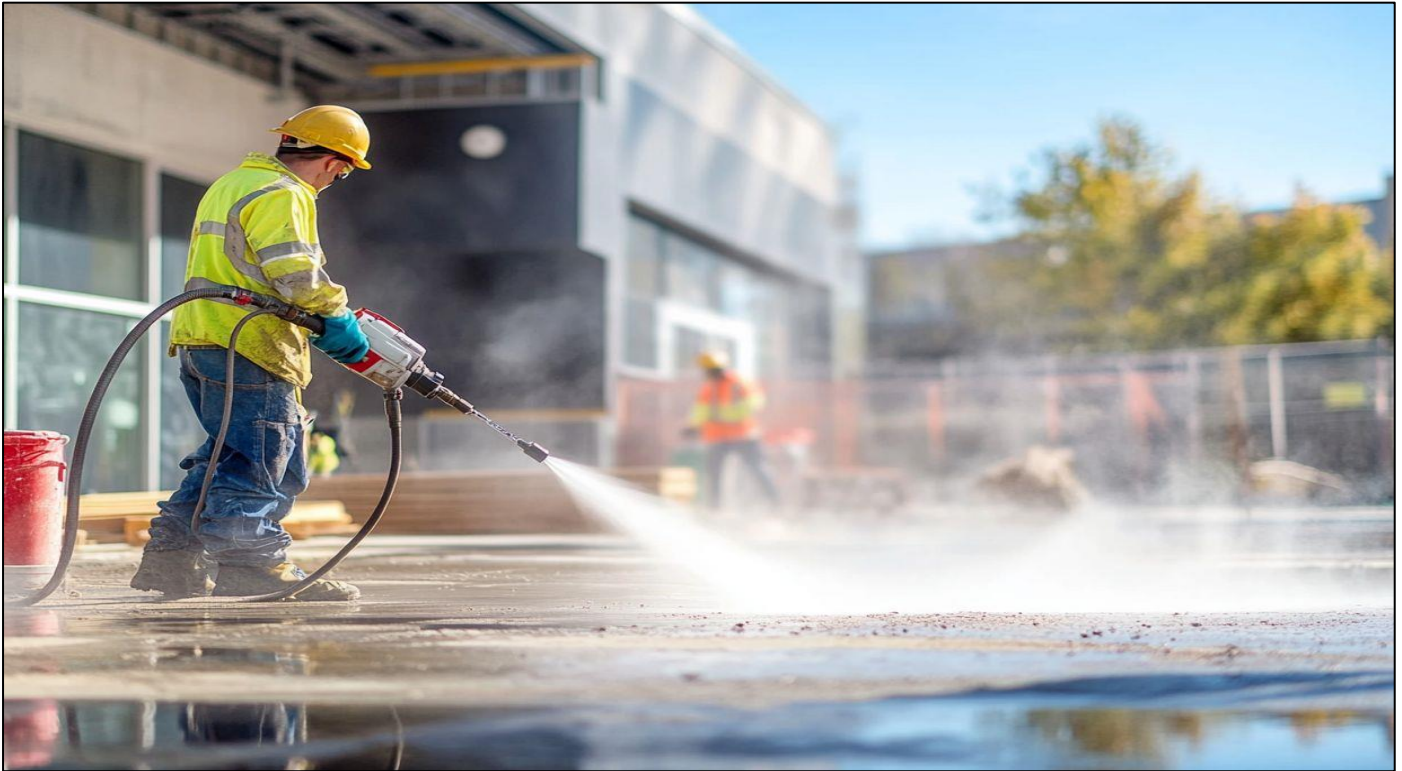
Fig 1 Applications of Pressure Washing for Post-Construction Cleaning (Peter, 2024)
