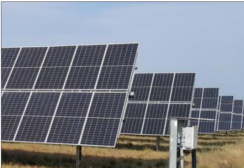
Fig. 3 Jinko solar model JKM580M-7RL4-V, 580Wp/unit
