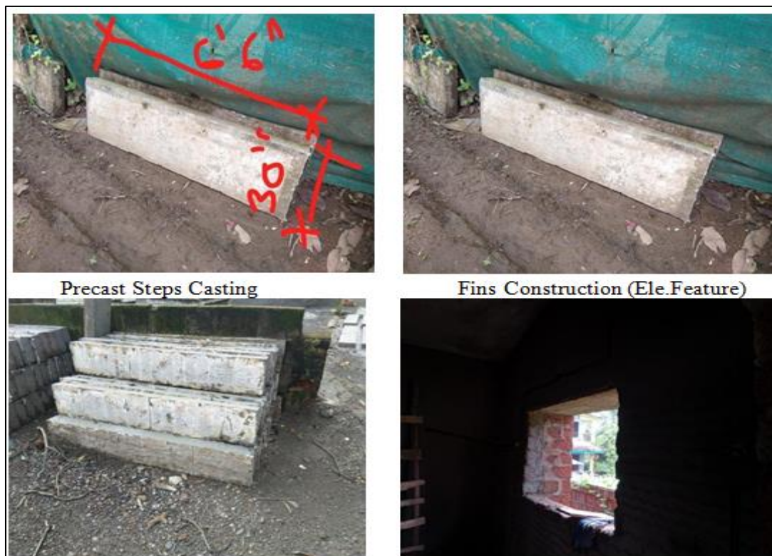
Fig 5 Showing Precast Elements on site Onsite
