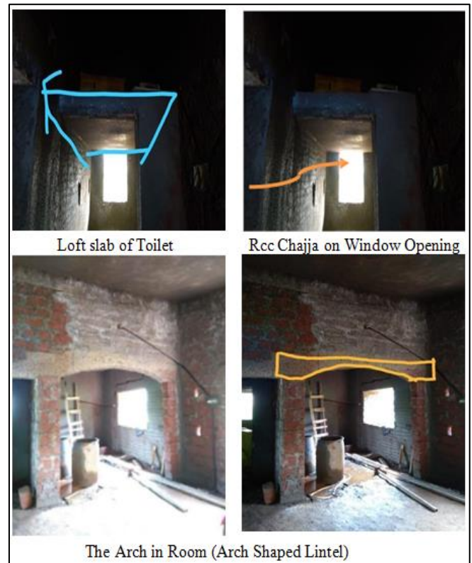
Fig 7 Construction with Partial Precast Elements
