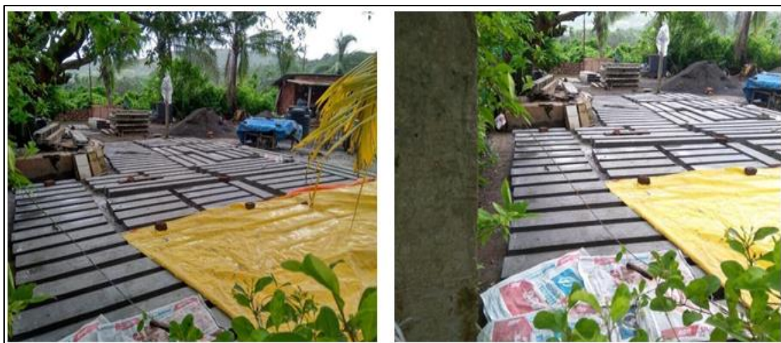
Fig 2 Images Showing Loft, Chajja, Slab casting
