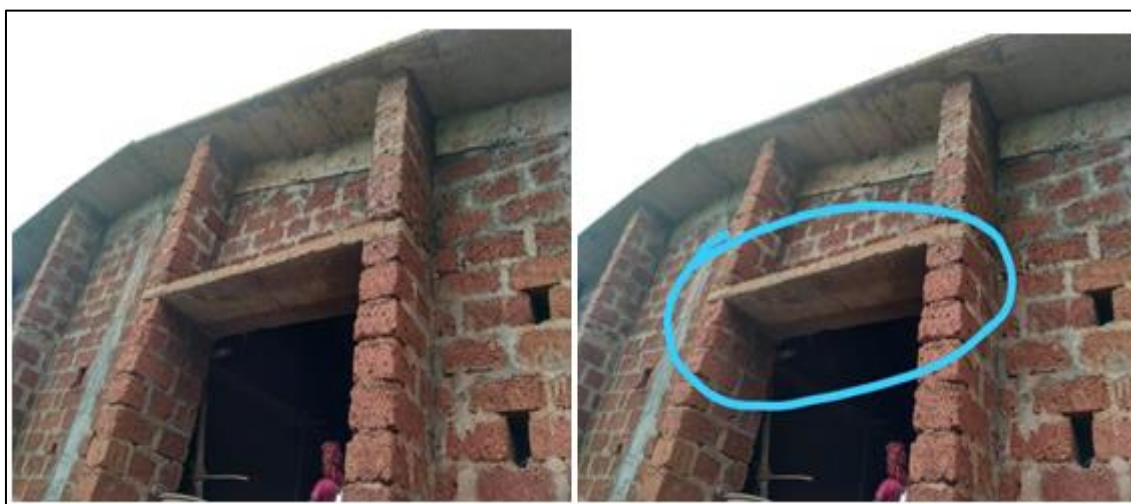
Fig 1 Precast Chajja Resting& Fixed Along with the Chira Stone
