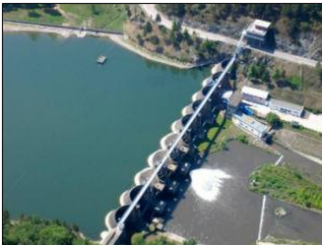
Fig 1 Dam and Accumulation Modrac
