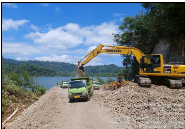
Fig 9: Provision of Materials and Work Tools at the Project Location
