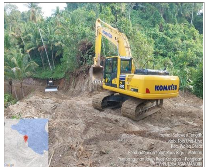
Fig 13: Dredging or Slope Repair
