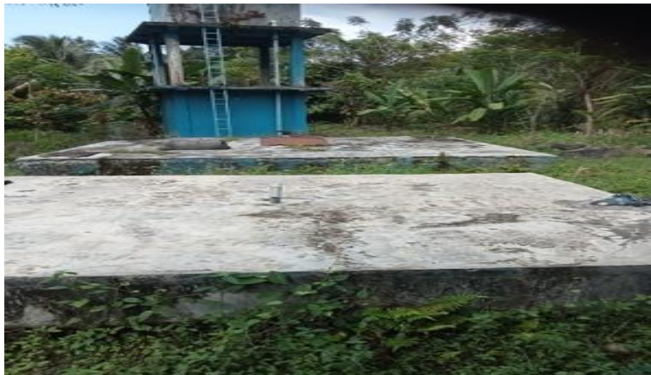
Fig. 3: Kajowou Water Treatment Plant and Storage Tank
