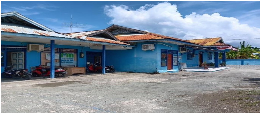
Fig. 5: Condition of the outside of the Water Treatment Plant Service Office and Soil Water Storage Tank
