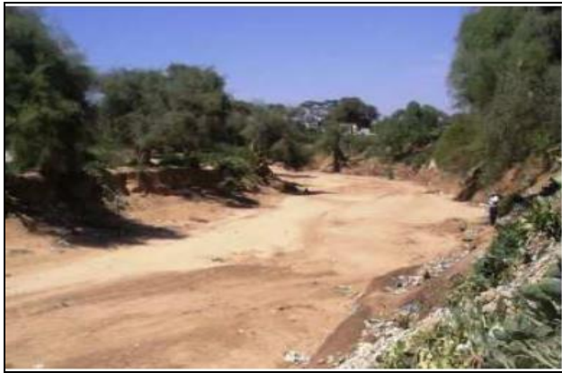
Fig 4: Person Stands on the Remains of Subsurface Dam [6]
