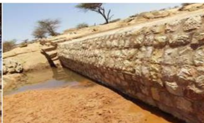
Fig 8(ii): AL HAYAT Dam front view
