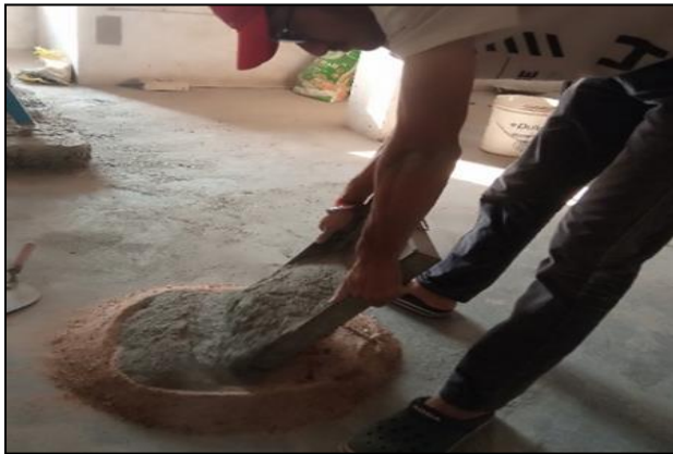
Fig 3: Concrete Mixing
