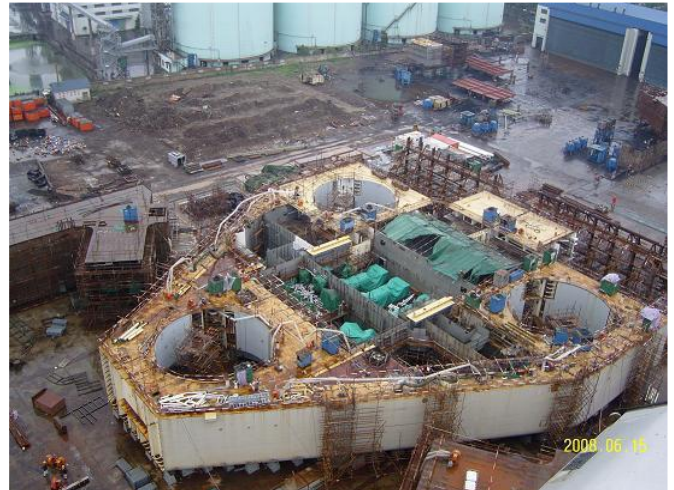
Fig 6 Early stage Construction
