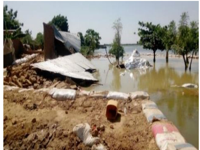
Picture 3 Maisons Collapsed Non-Durable Houses Source: Gassina P., September 2020
