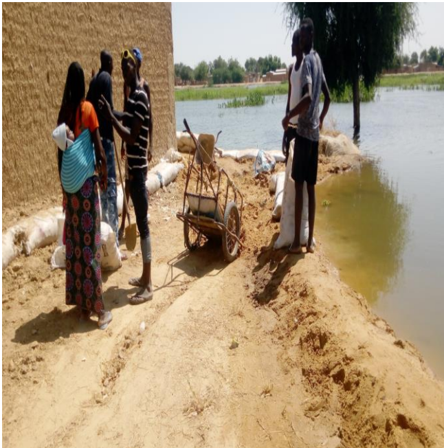
Picture 5 Erection of Embankments Around Housing Source: Gassina P., September 2020
