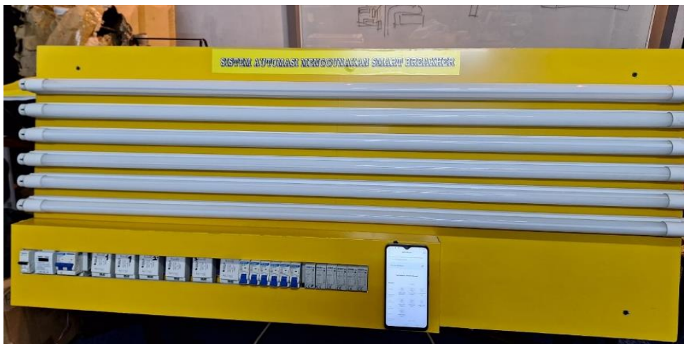
Fig. 6: Real Application From Smart Breaker Control
