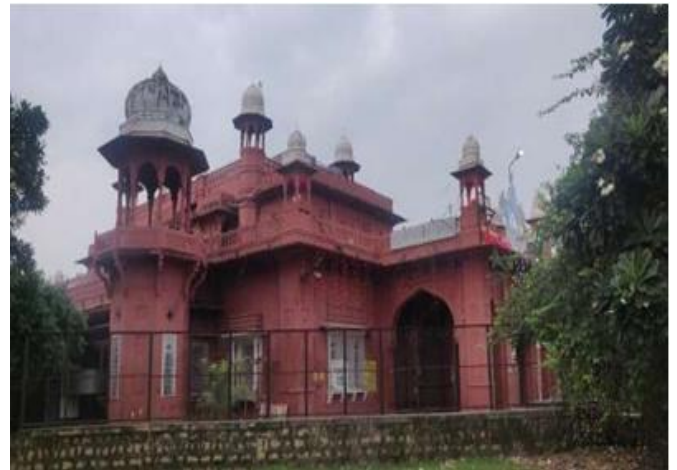
Fig 13 Edward Museum Architectural Style: Islamic Style Built -1908 Built – 1898
