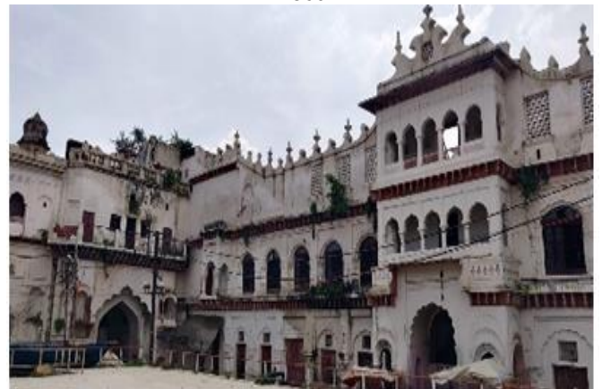
Fig 9 Moti Mahal Architectural Style: Islamic Style Built - 1874
