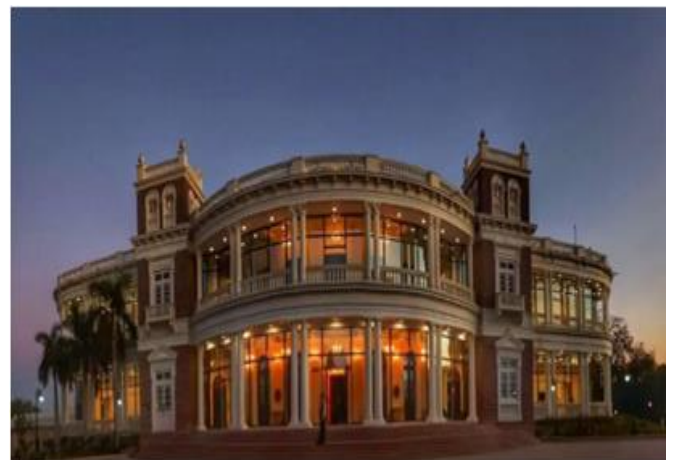
Fig 14 Minto Hall Architectural Style: Indo Colonial Style And Nawabi Style Built -1909
