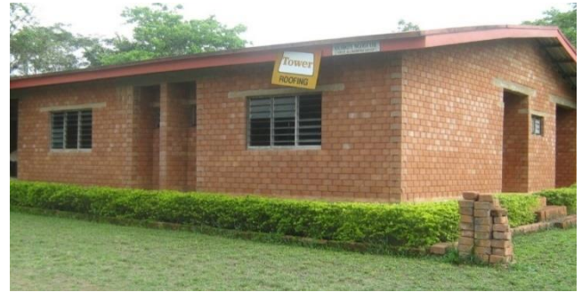
Plate2: An example of a compressed stabilized laterite bricks building in Ota, Ogun State Nigeria.
