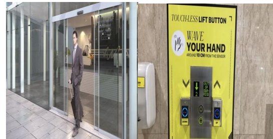
Fig. 18: The use of hygiene technologies to control cleanliness of the room and the users' health – Automatic doors and touchless lift buttons (Source: Google)
