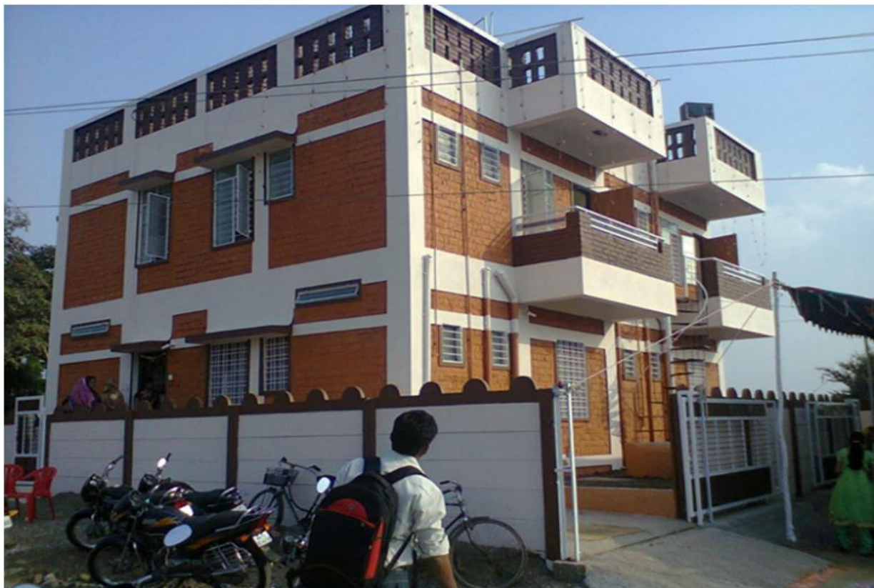
Plate 5 Two-Storey Building using Bamboo and Nominal Rods as Reinforcement. Source: https://timesofindia.indiatimes.com/city/nagpur/pwd-allows-bamboo-as-mainstream-construction-material/articleshow/79189140.cms
