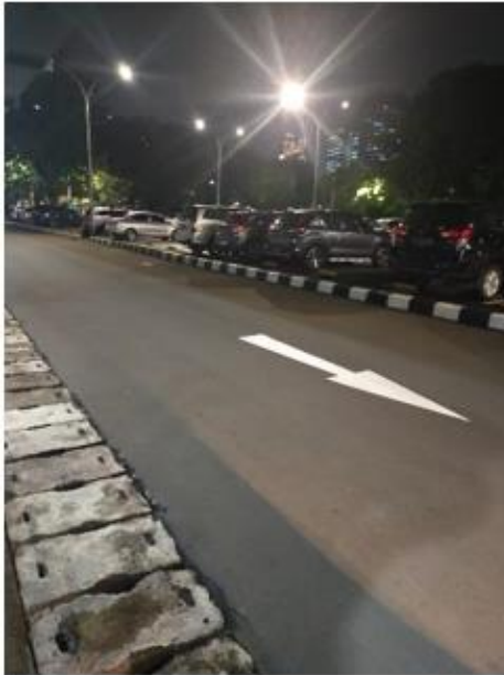
Fig 2:- Parking Area and Gambir Station Street
