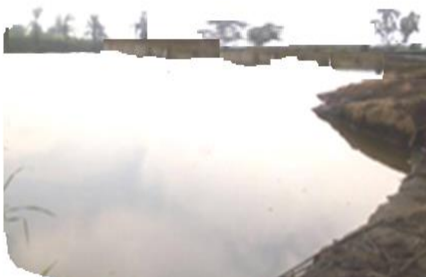
Fig. 2: Unlined Depot Waste Water Discharge Pit
