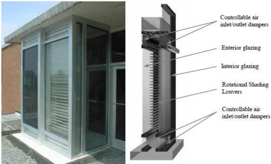
Fig 1:- Smart façade system installed in the College of Architecture building, Georgia Institute of Technology
