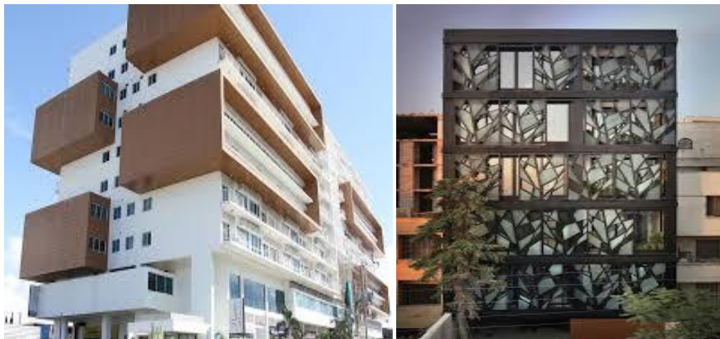
Fig. 1: Different building facades (Source:www.kaercher.com, 2021)
