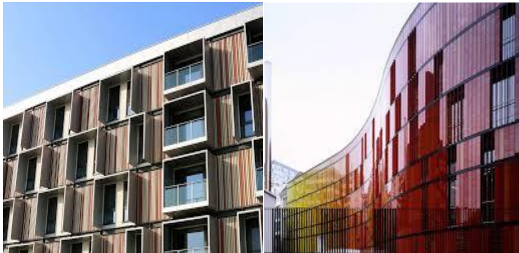
Fig. 2: Different Building Facades (Source:www.kaercher.com,2021)
