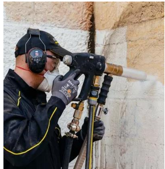
Fig. 5: Water Pressure Hose Used In Façade Cleaning
