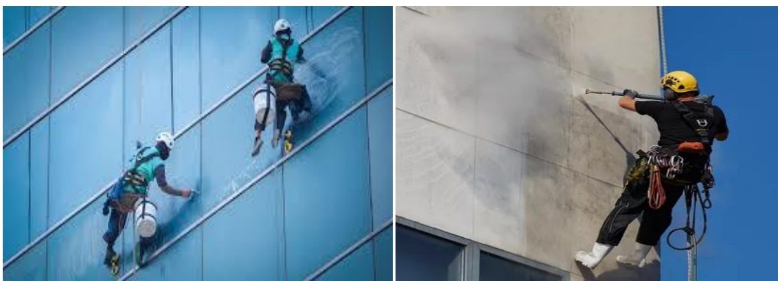
Fig. 3: Window Cleaners And Steam Hose Used In Façade Cleaning (source:www.ranpc.com,2022)
