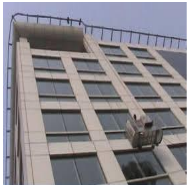
Fig. 8 :Automated Façade Cleaning Device
