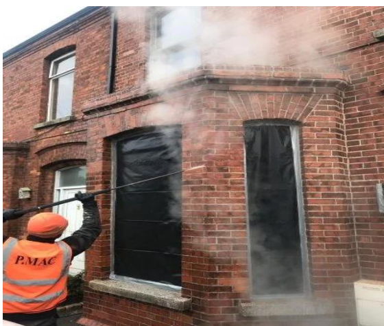
Fig. 4: Steam Hose Used In Masonry Façade Cleaning
