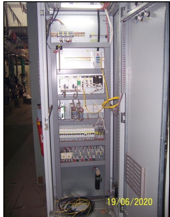
Fig. 10: Main PLC panel internal arrangement
