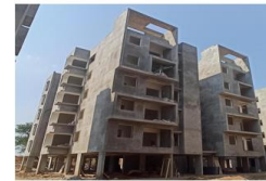
Exterior cement work done ( Block A )
