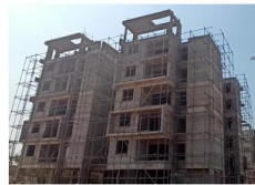
Brickwork in 5 th floor ( Block C )
