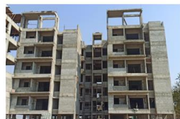
Brickwork completed ( Block D )
