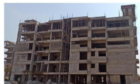
Slab under construction ( Block E )
