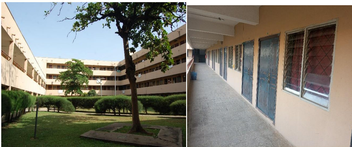
Fig. 6: Use of Deep Verandas and Balconies as Shading Elements
