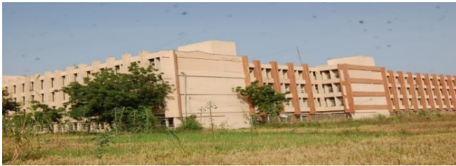
Fig. 5: Shading devices of the FSCB, building
