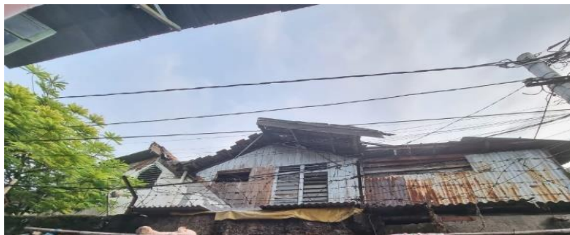
Fig. 4: Side view of the case study building
