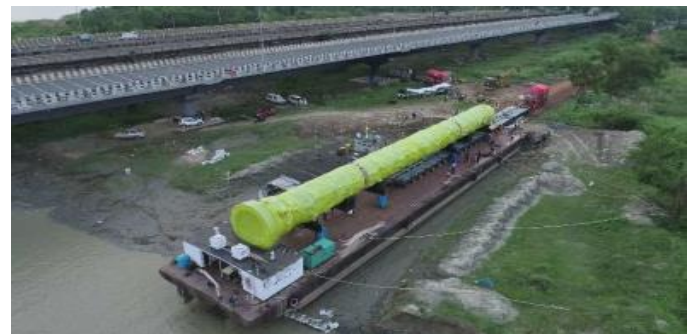
Fig. 6: Roll off by a Modular transporter [4]
