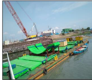
Fig. 4: Lifting from barge to trailer at LOLO Jetty
