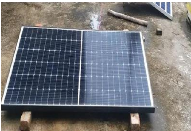
Fig. 13 Solar panel used to charge the battery pack of 24 V, 10 Ah
