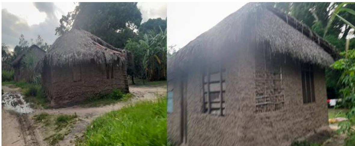
Fig 3 Mud Walls with Grass-Thatched Houses Source: Field Survey, 2022
