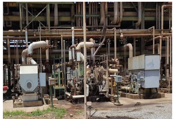
Fig. 1: KRPC HP Pumps
