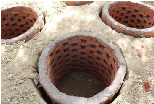
Fig 2. Semiconstructed pits.
