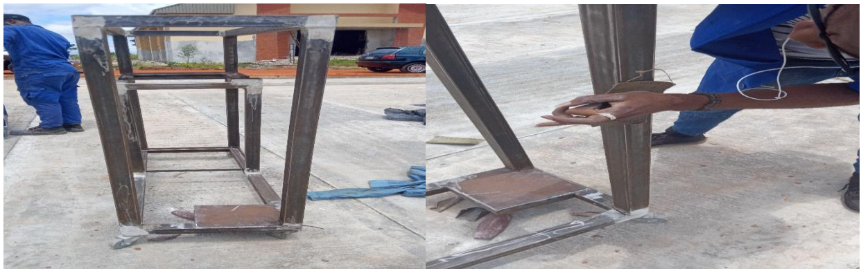
Plate 3: Grinding and Smoothing Operations
