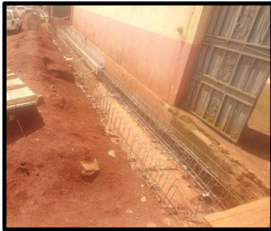
Photo 4 and 5: Gutter construction in Bamendzi-ville A
