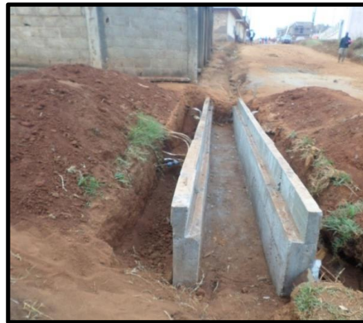
Photo 4 and 5: Gutter construction in Bamendzi-ville A
