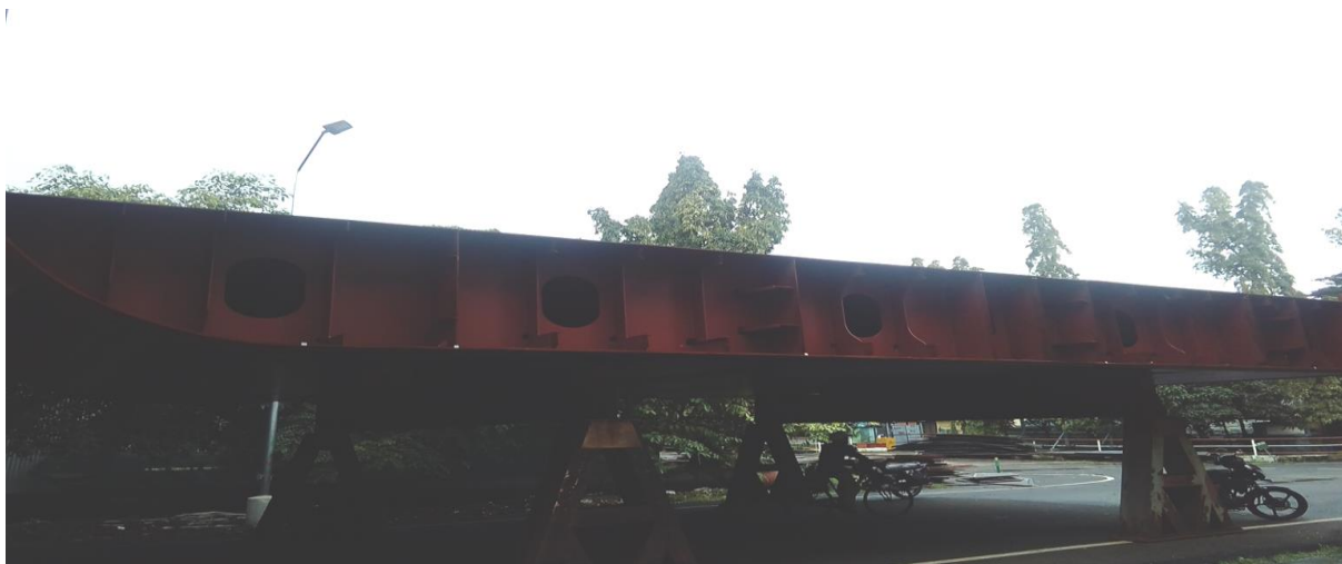
Fig 3:- Blocks place with retro-reflector targets for taking measurement.
