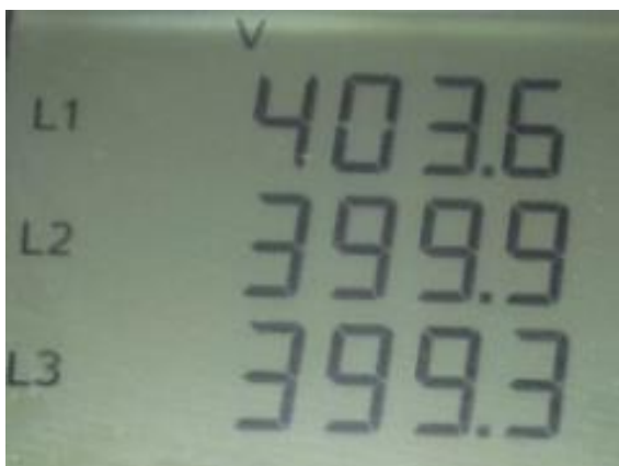
Fig 7:- Voltage of L1, L2, and L3 on Trial-1
